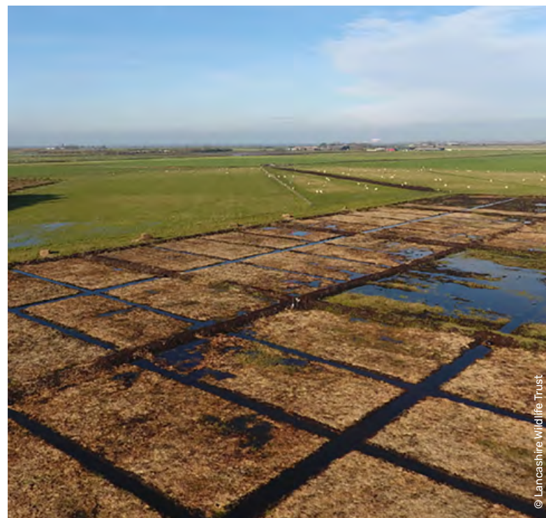
Figure 19: The Winmarleigh Carbon Farm. The newly created grid pattern of banded cells, irrigation ditches and channels, with a protective layer of straw covering the newly planted plugs of Sphagnum moss (November 2020).
